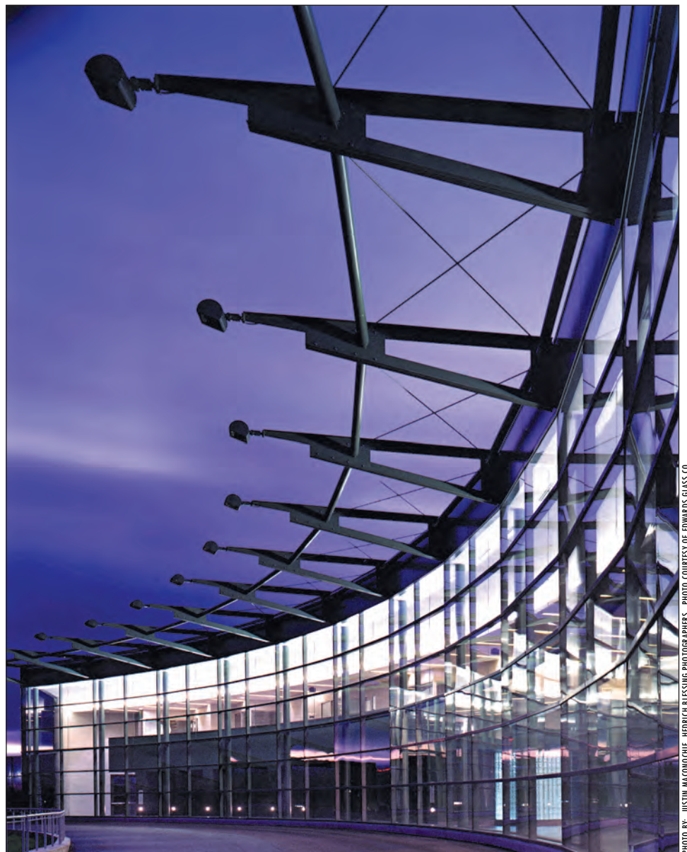
High-performance Low-E glass and a custom anchoring detail shape this stunning wall of glass that offers a commanding view of the football field from the lobby interior.
