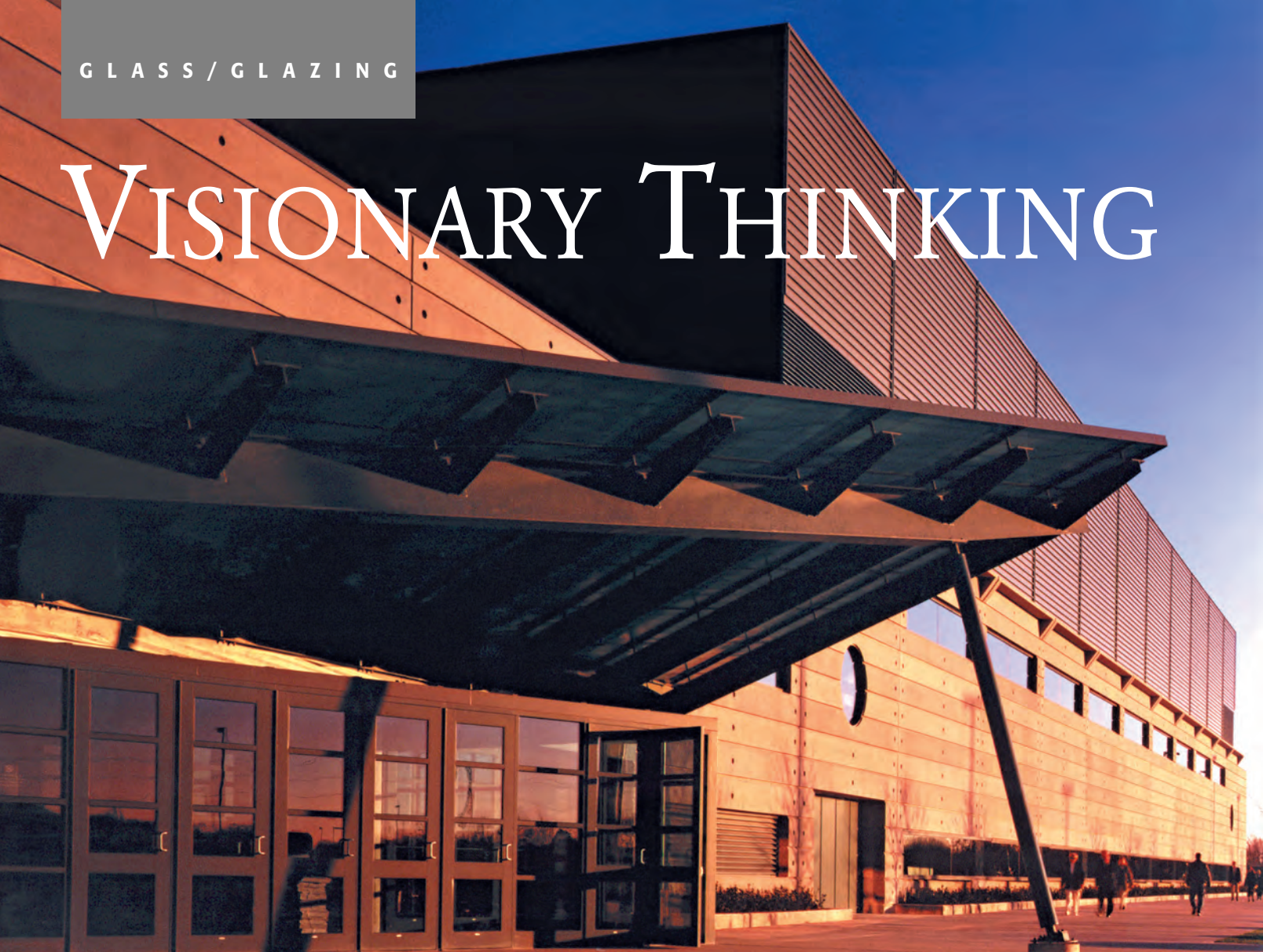
A triangular canopy and a skewed glass vestibule mark the distinctive entrance to the EMU Convocation Center.
